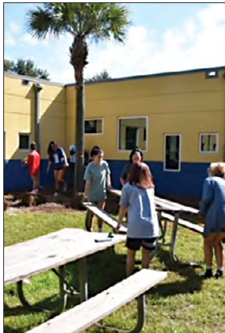
Work on the outdoor classroom taking place on the first day.
