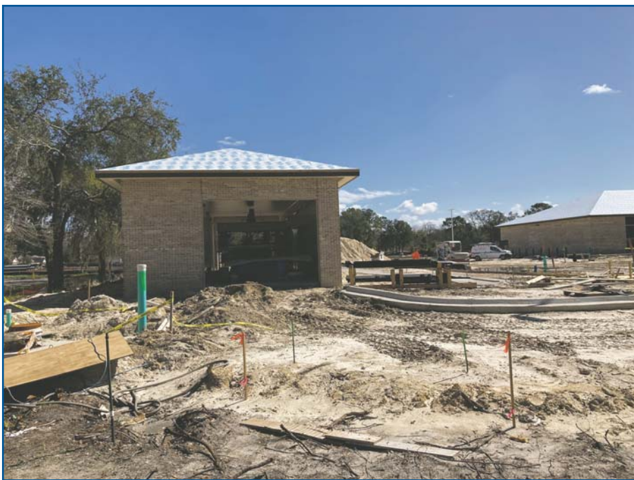
Photos courtesy Martie Thompson The car wash under construction.
