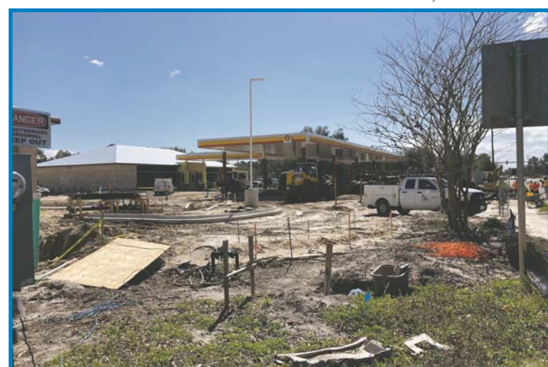
The Daily's on San Jose Boulevard under construction.
