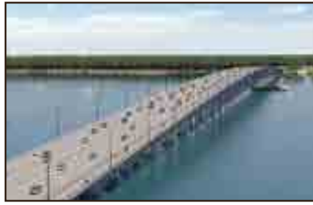
Photo courtesy Florida Department of Transportation The Florida Department of Transportation will begin construction on a new bridge over the St. Johns River in fiscal year 2022.
